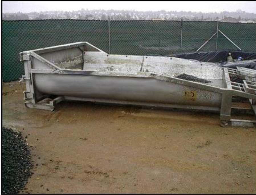
Photograph 5 Typical Washout Facility
