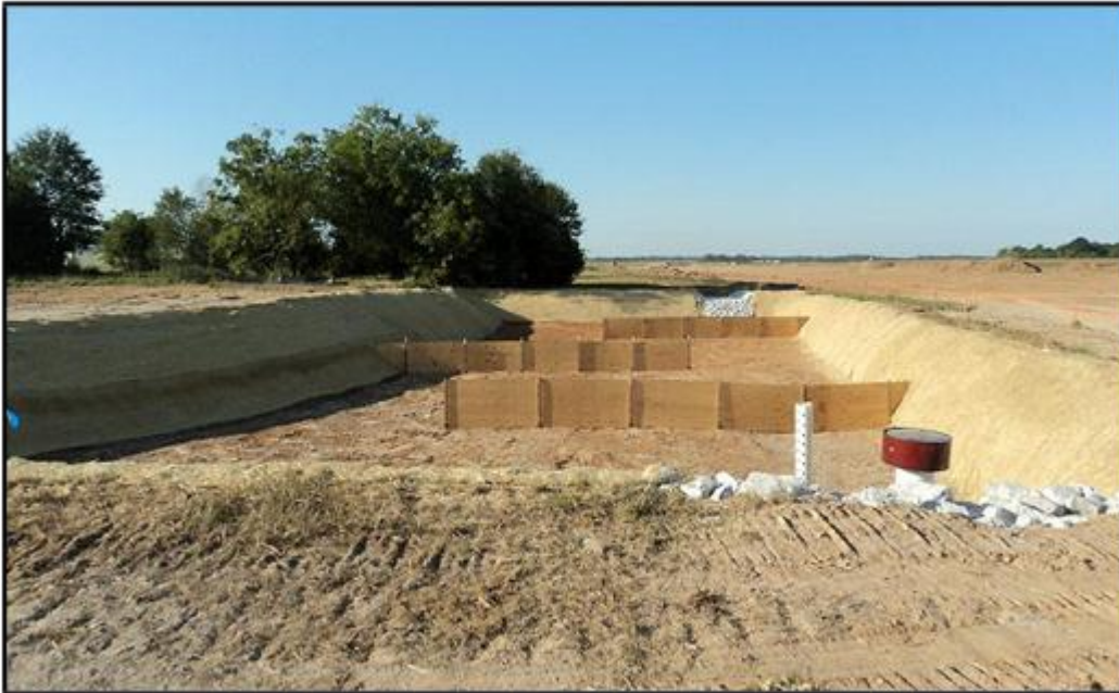
Photograph 1 Typical Diversion Channels in a Settlement Pond
