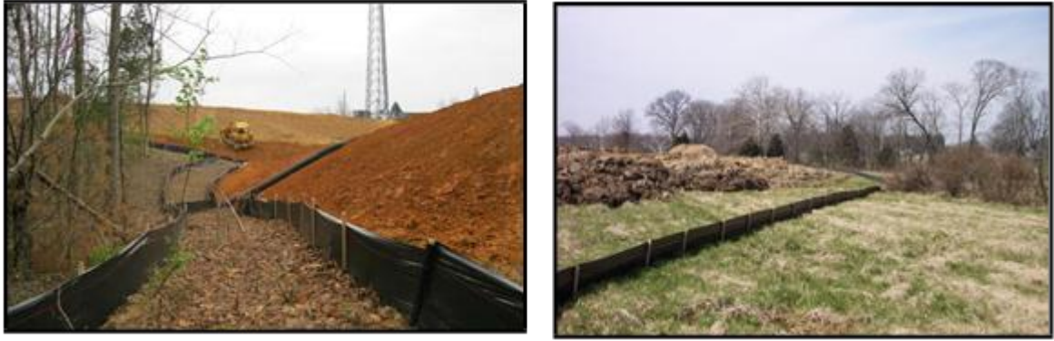
Photograph 2 Typical Silt Fence Usage
