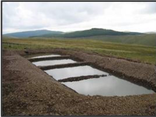
Photograph 4 Typical Settlement Pond / Lagoon
