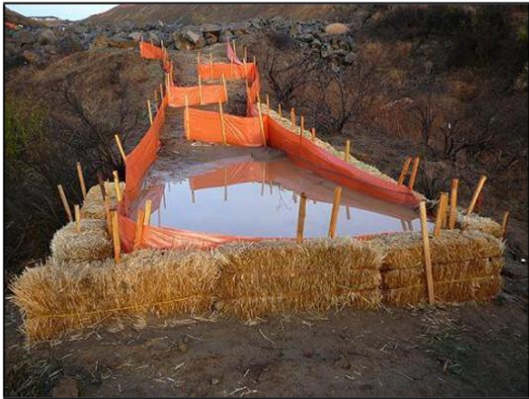
Photograph 3 Typical Silt Fence Adjacent to Road Cutting
